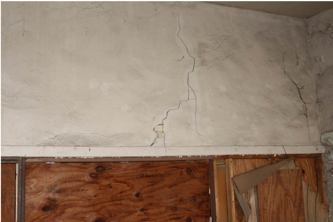
Photo No. 14: On the south side of the house, it appeared that the lower half of an interior masonry wall had been removed, was supported with wood stud framing, and appeared to be sagging. (2 of 2)
