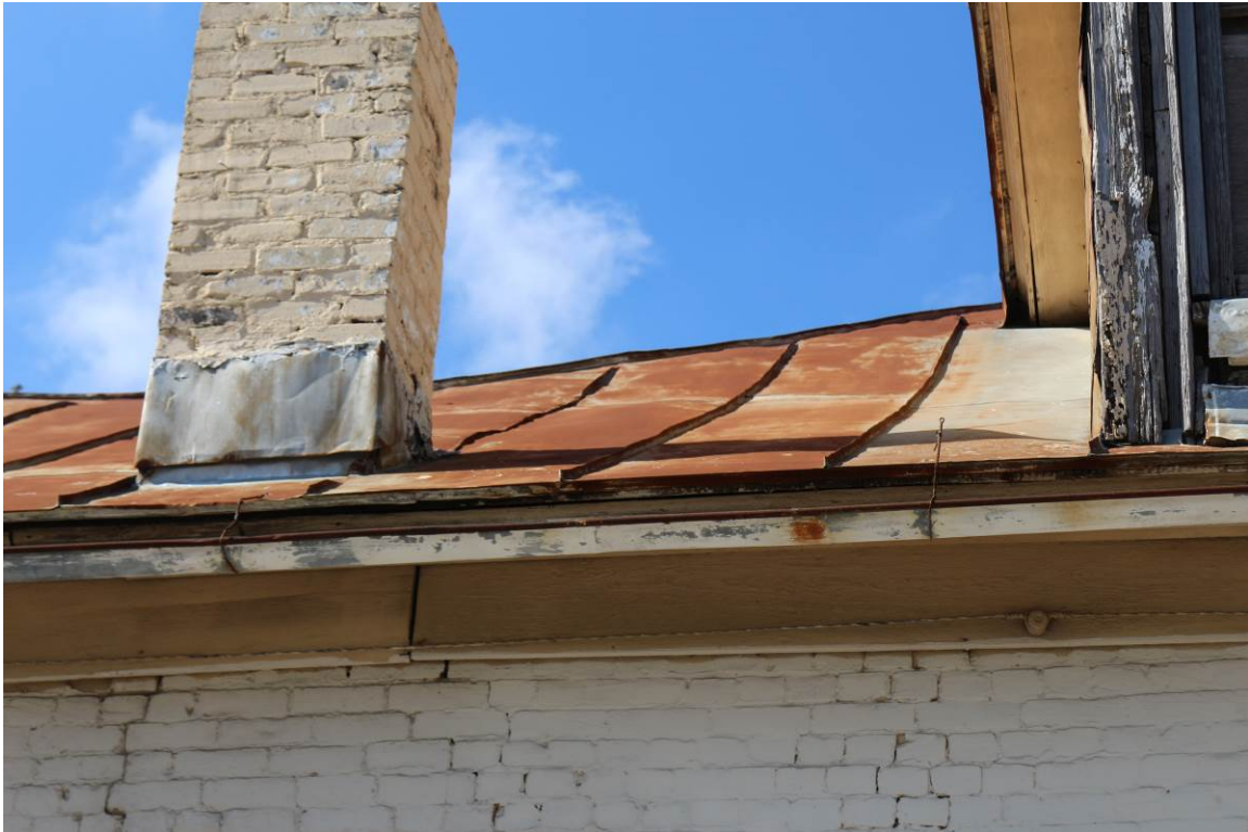
Photo No. 15: There were areas of sagging roof.
