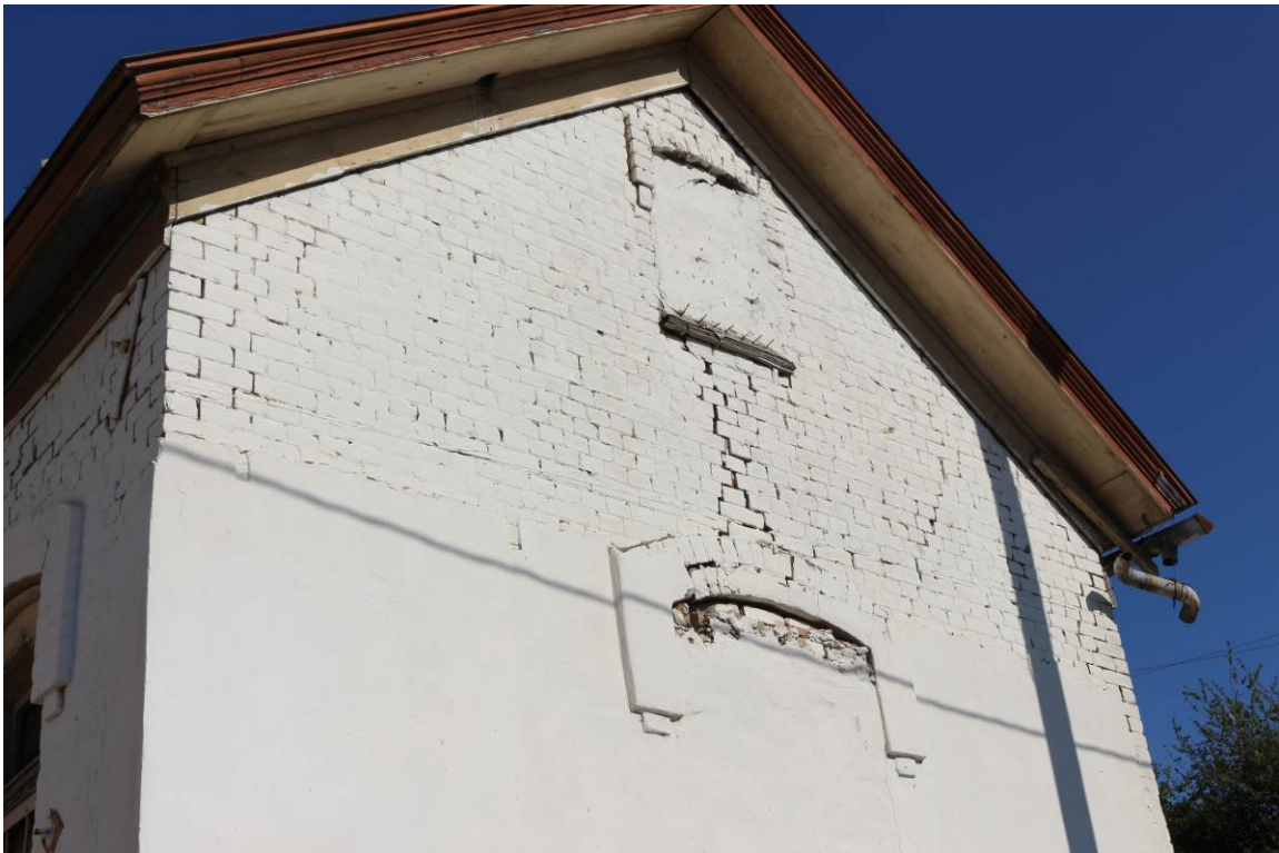
Photo No. 10: There were numerous and widespread vertical and diagonal cracks and separations in the walls of the building. (1 of 2)
