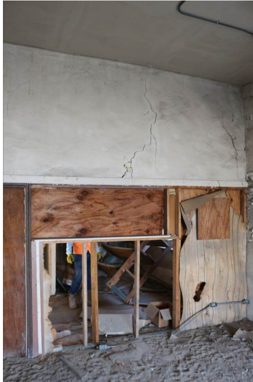
Photo No. 13: On the south side of the house, it appeared that the lower half of an interior masonry wall had been removed, was supported with wood stud framing, and appeared to be sagging. (1 of 2)
