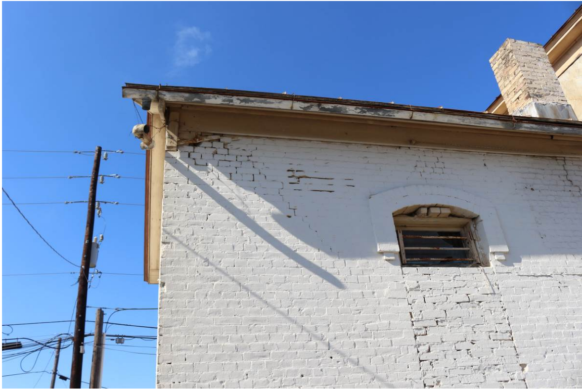
Photo No. 11: There were numerous and widespread vertical and diagonal cracks and separations in the walls of the building. (2 of 2)
