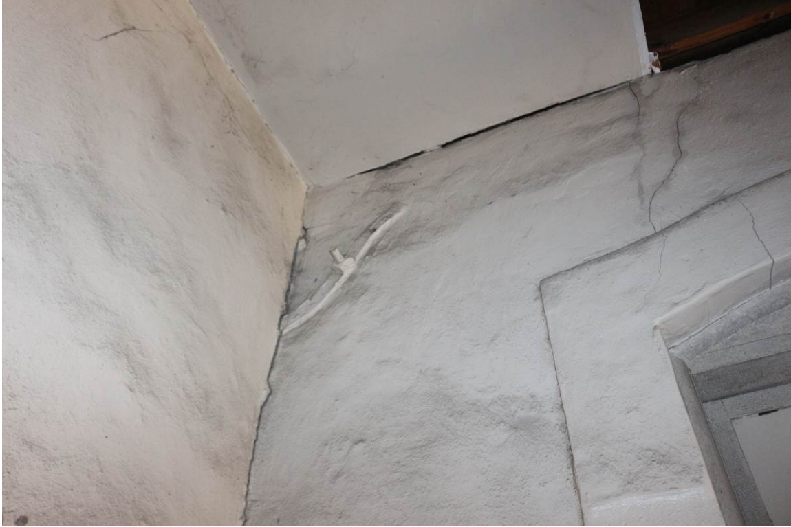
Photo No. 9: There were rods with bearing plates spanning from wall to wall, across entire rooms, observed at several corners of the building. (2 of 2)
