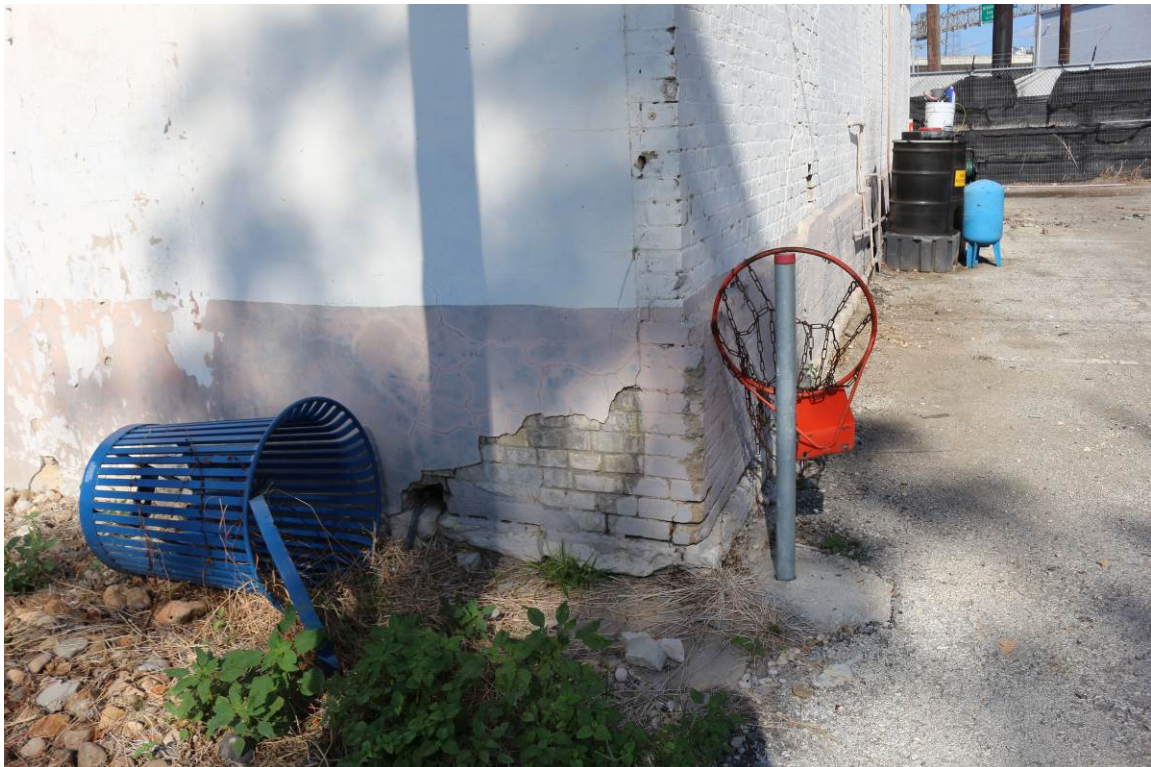
Photo No. 12: It appeared as though the top of the foundation footings dipped down at the corners of the building.
