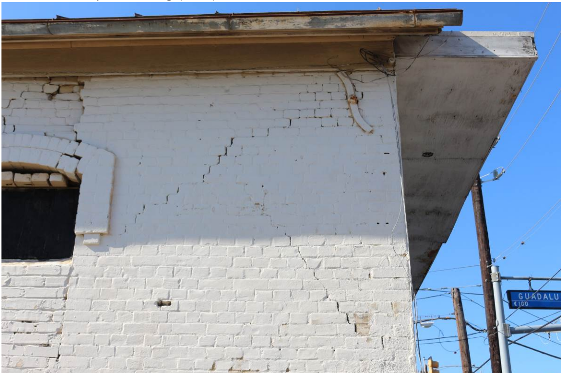
Photo No. 8: There were rods with bearing plates spanning from wall to wall, across entire rooms, observed at several corners of the building. (1 of 2)
