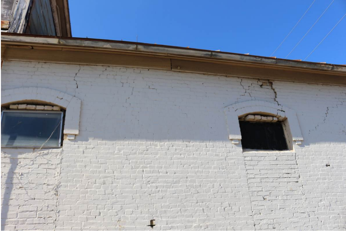
Photo No. 7: There was missing mortar, cascading and/or sagging masonry, cracked and misaligned lintels, and localized out-of-plane buckling. (2 of 2)
