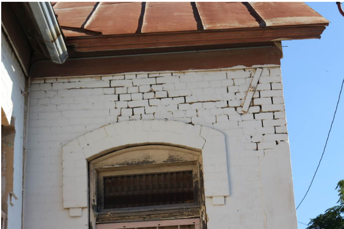
Photo No. 6: There was missing mortar, cascading and/or sagging masonry, cracked and misaligned lintels, and localized out-of-plane buckling. (1 of 2)
