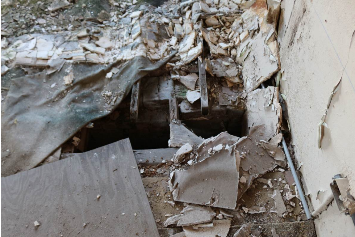
Photo No. 17: On the first floor, approximately 40% of the flooring was rotted or missing entirely
