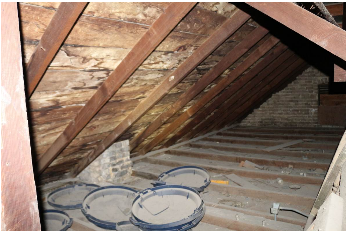
Photo No. 16: There was widespread rot and possible biological growth on most of the roof framing and decking.
